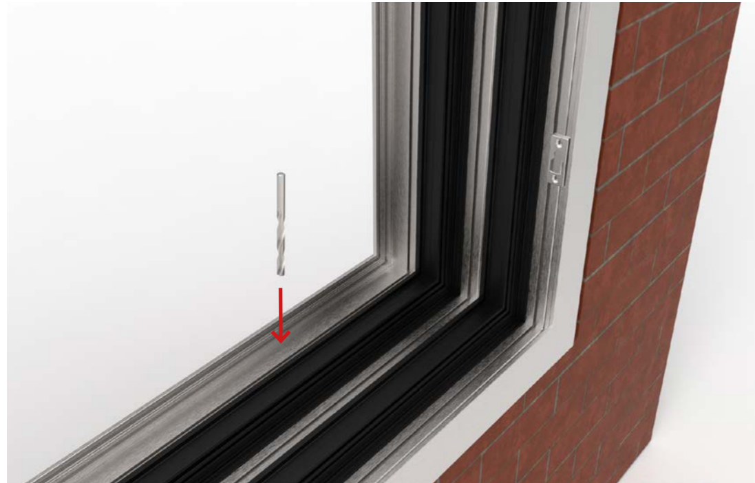
3 Drill an appropriate sized fixing hole through the frame. This should be no more than 200 mm from the external corner of the frame.
